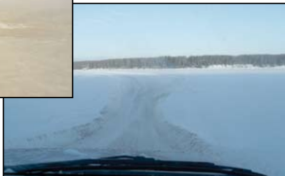
Entrance on to the completed ice bridge.
